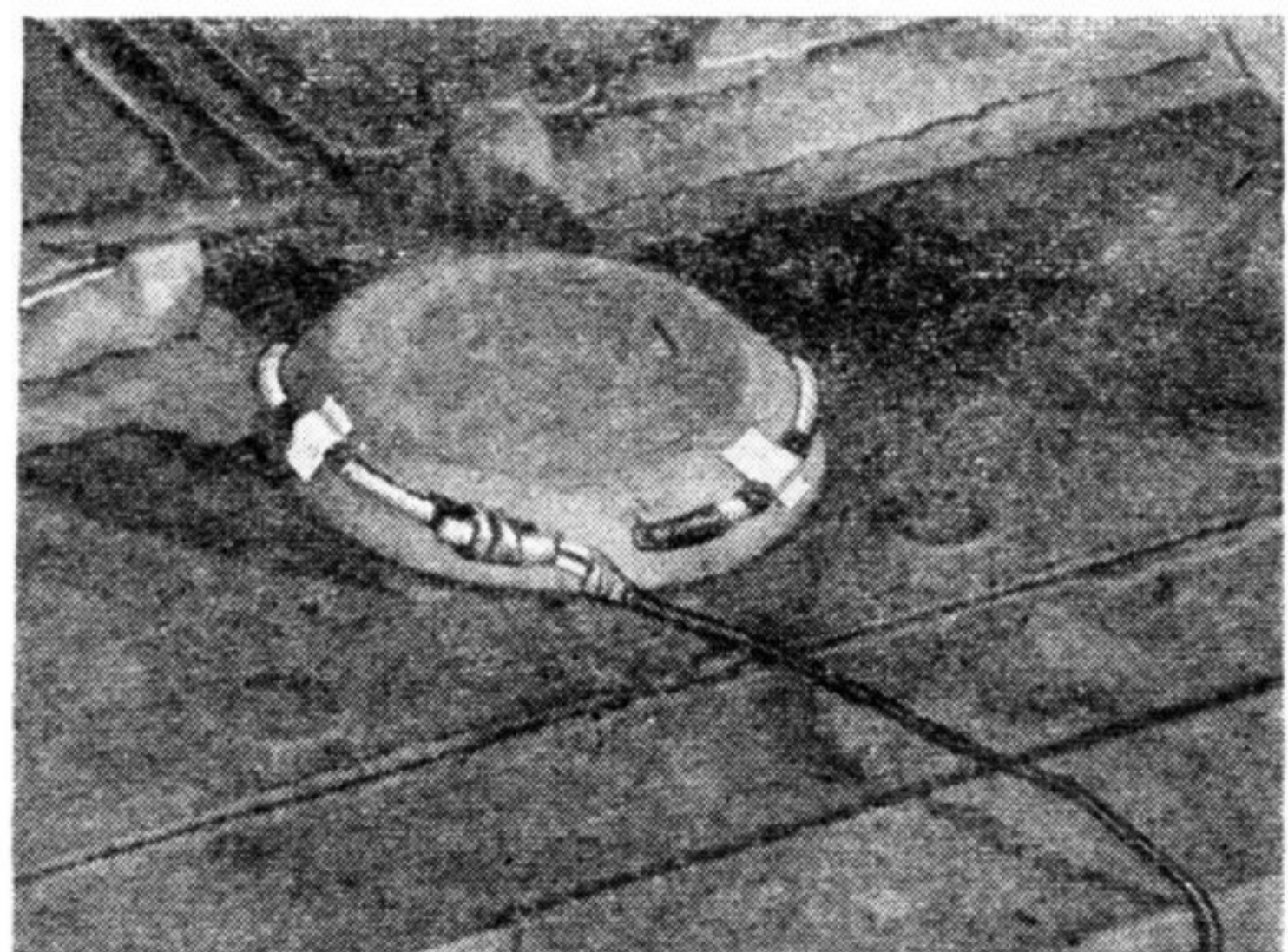
OPERATION 45. Cordtex fitted to front fan ventilation dome.
